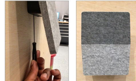
Fig.4: Secure fixture to mounting plate.
