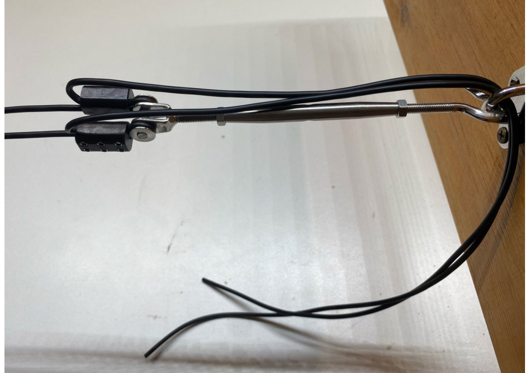
Fig 7.1 Run power cables to power supply.
