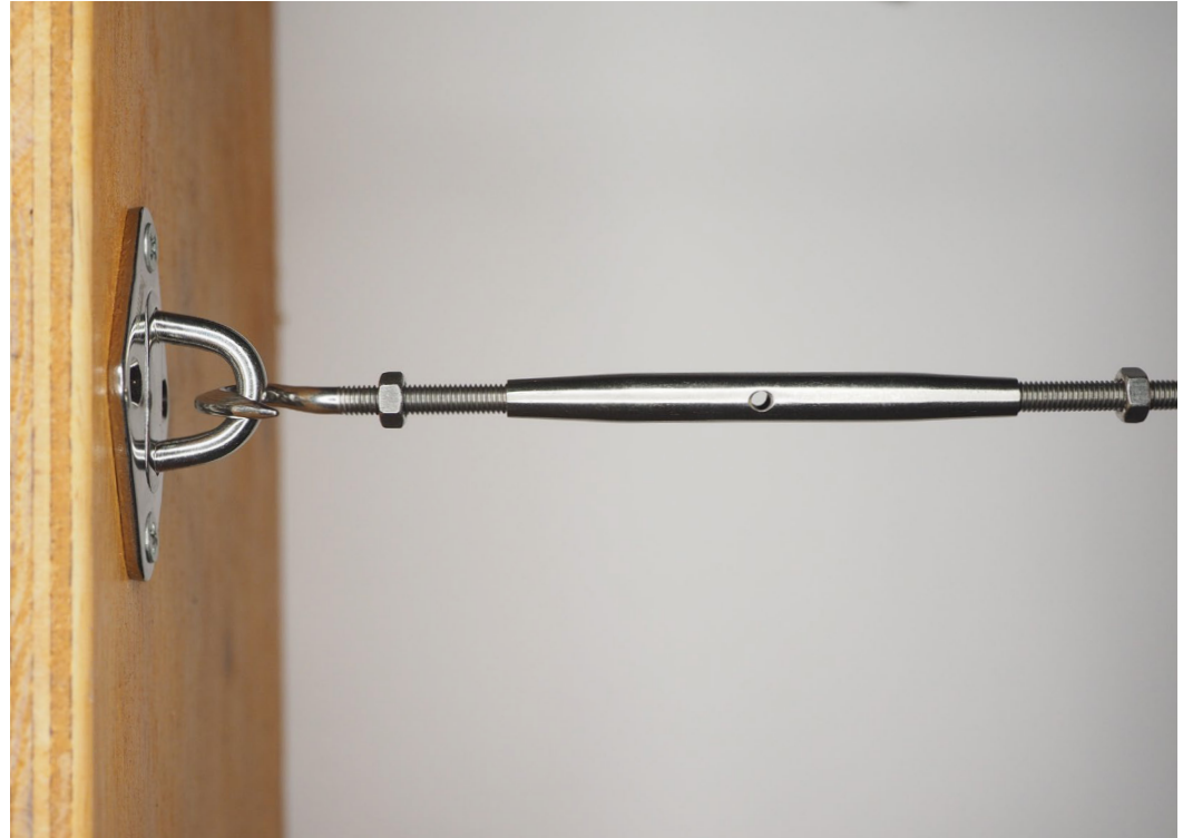
Fig 3.1 Reattach turnbuckles to each mounting device ensuring they are at their fully extended state as pictured.
