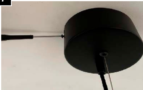
Fasten canopy screw to the canopy.
