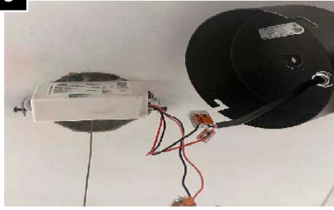
Connect LED + and LED - wires from fixture to LED + and LED - wires from driver. Note: Wire leads from WEP shade may be Black / White. Reference Labels. DO NOT WIRE TO LINE VOLTAGE.
