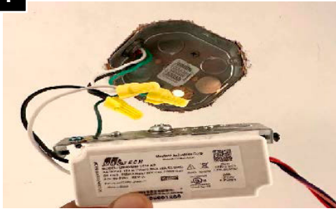
Remove driver bracket from canopy. Connect line voltage and ground wires to building wires. (If necessary, connect dim wires)
