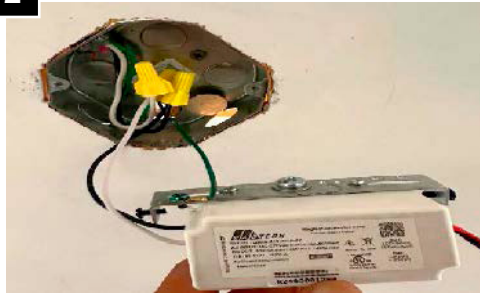
Place line voltage wires inside junction box.
