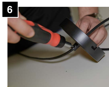
6 After adjusting cord length, tighten set screw on canopy.
