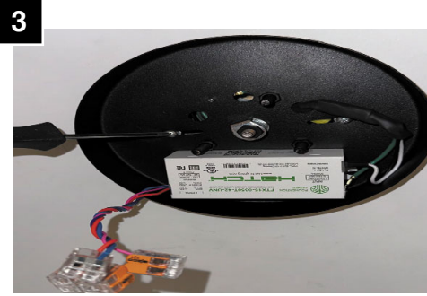
3 Fasten canopy to junction box using j-box screws (by others).
