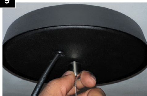
9 Thread cable coupler to canopy to suspend fixture.
