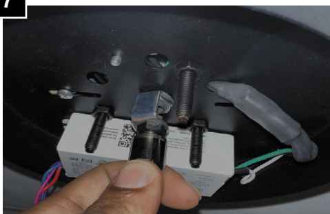
7 Unthread aircraft suspension coupler while holding fixture with opposite hand or with additional help.
