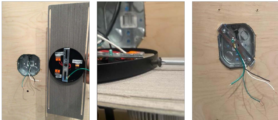
Fig.1a: Wiring for junction box to fixture.
