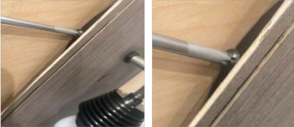
Fig.3: Secure canopy to mounting brackets using canopy screw.
