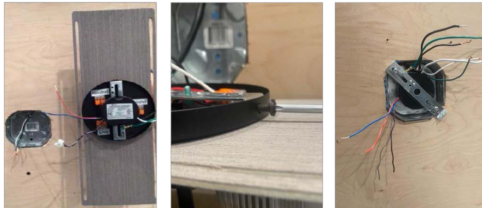
Fig.1b: Wiring for junction box to fixture.
