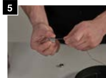
Twist off end cap from cable coupler and feed aircraft cable.
