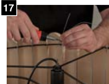
17 Tighten both screw of strain relief and adjust aircraft cable length as needed. Cut loose aircraft cable if necessary.
