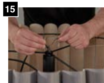
Loop same end of aircraft cable through balancer.
