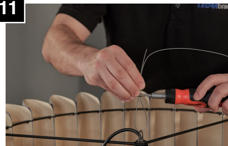
Tighten both set screws and cut loose aircraft cable if necessary.
